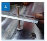
Fit universal fixing bracket with roof sealing washer and screw.
