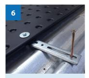
Place collector on bracket and attach using nut and washer. ON LEFT AND RIGHT SIDE OF PANEL USING CENTRE HOLE.
