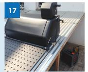
Fit piping via conex fittings and clamping into solar connectors.
