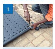
Attach solar connector and stopend using supplied clamps.
