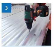
Locate batton where panel will be fixed on. Drill 6mm hole on high end of roof.
