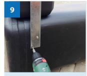
Fit cistern tank onto geyser using supplied tek screws.
