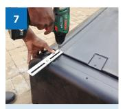
Fit universal fixing bracket to the bottom of the geyser using supplied tek screws.
